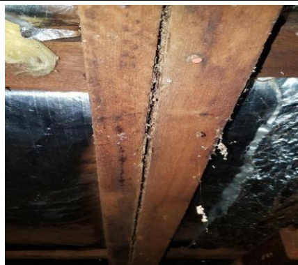
Workings in the roof space with no structural damage noted in the accessible areas checked.
