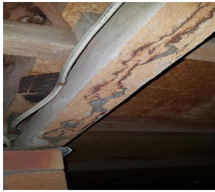
Workings in the subfloor with no structural damage.
