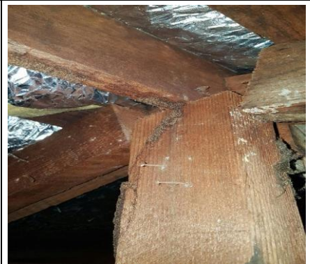
Workings in the roof space with no structural damage noted in the accessible areas checked.
